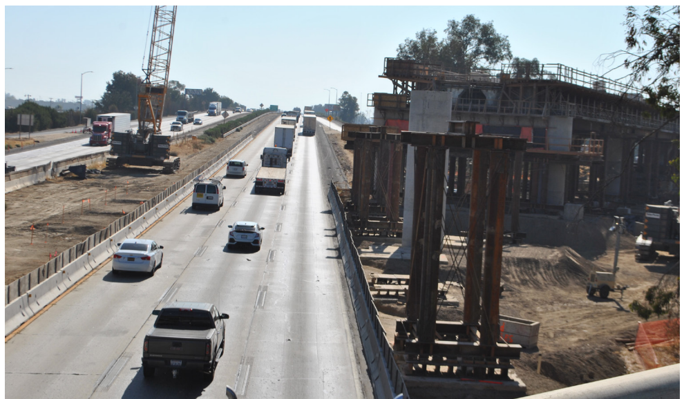
California High-Speed Rail Cedar Viaduct under construction in 2019 – photo from CAHSRA
